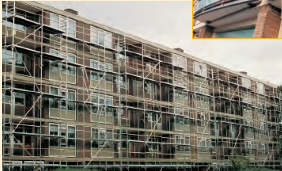
35 flats. Balcony extension by fitting prefab balcony floors. The built-in balcony floors are raised with shot-concrete and equipped with anchors from the scaffold brackets at wall side. After removing all brackets on balcony height, the prefab floors are hoisted inbetween scaffold and wall and equipped with haul rods and guardrails. The scaffold is composed from 1.8 and 2.5 m length with 2.0 and 2.8 m platform height combinations.
