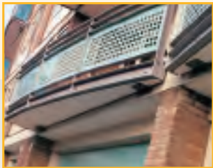
35 flats. Balcony extension by fitting prefab balcony floors. The built-in balcony floors are raised with shot-concrete and equipped with anchors from the scaffold brackets at wall side. After removing all brackets on balcony height, the prefab floors are hoisted inbetween scaffold and wall and equipped with haul rods and guardrails. The scaffold is composed from 1.8 and 2.5 m length with 2.0 and 2.8 m platform height combinations.
