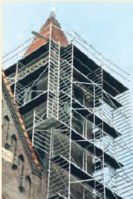
Convent. Replacing roof-slats at the spire. The scaffold may not support on the church roof below; therefore a free-hanging construction in front of the side wall, connected to tower sections alongside the front and back wall. Tower sections: 2 x 2.5 m extended with semi-open intermediate frames. Total height 25 m.
